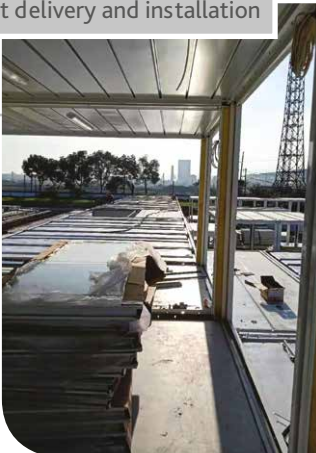
Fast delivery and installation
